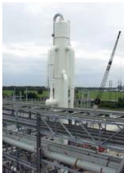
Right: Jet-Vac 2100 ton three stage water chilling system
